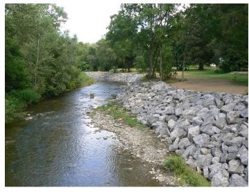
530 feet of streambank stabilization on Cattaraugus Creek
