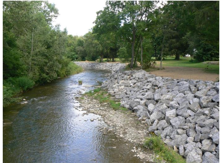
530 feet of streambank stabilization on Cattaraugus Creek
