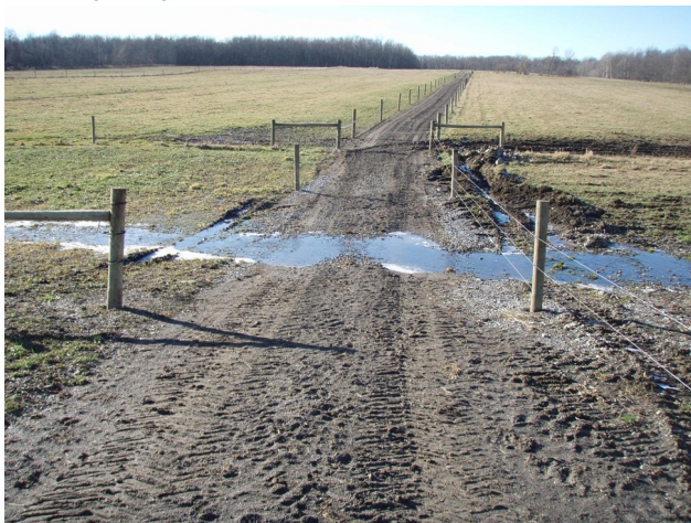
Stabilized stream crossing with animal walkway
