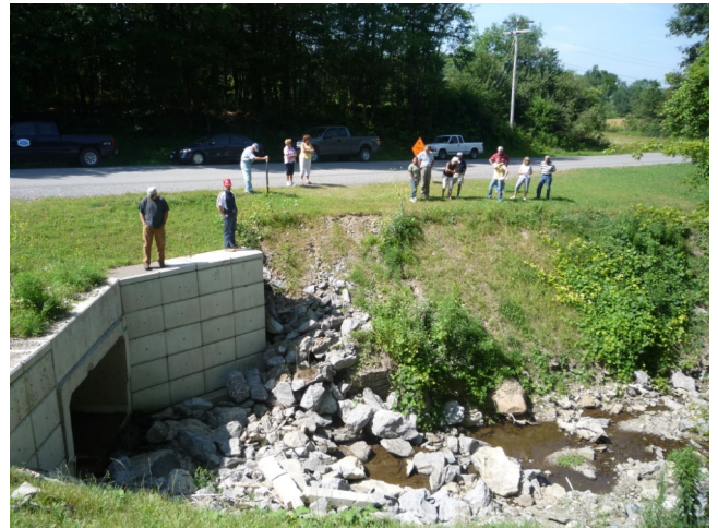
Culvert Replacement and Bank Stabilization on Cascade Rd. in Attica, NY.
