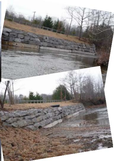
**Top Left** - Streambank stabilization to remediate an exposed water line in the Town of Attica, NY.
