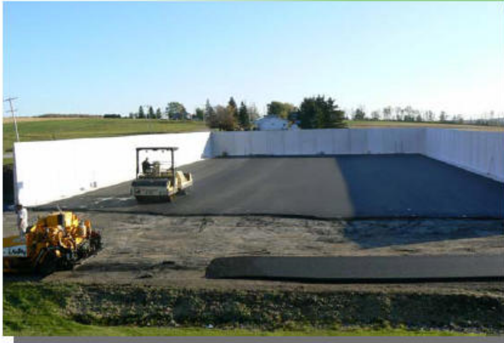
Friendly Acres Asphalt Bunker Silo & Leachate Collection System in Attica.
