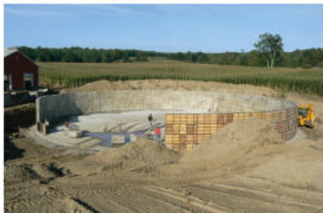
Concrete Manure Storage at Sally Tarey - Rickard's Farm In Pike.
