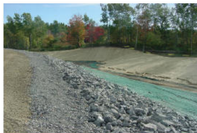
Erosion & Sediment Control at former ETE Sanitation Landfill site in Gainesville.
