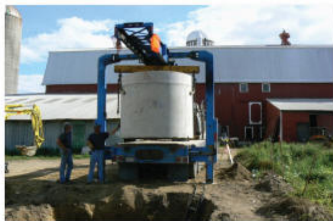
EQIP Milkhouse Wastewater Tank at Perl Valley Farm In Eagle.
