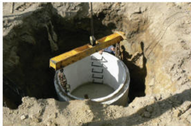
Bottom section of manhole being placed and leveled.
