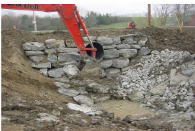
Culvert Stabilization on Exchange Street in Attica.
