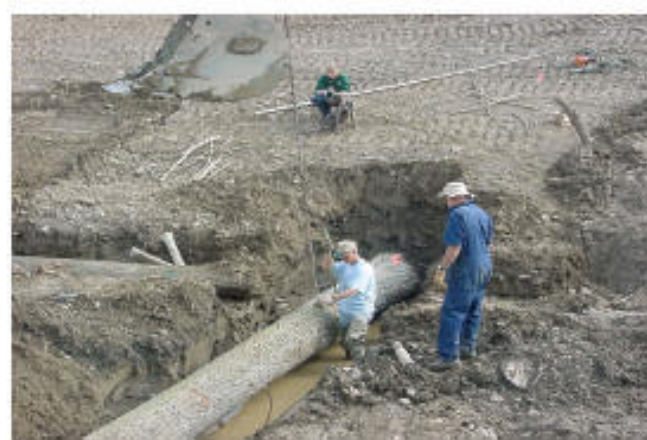
Installing Log Grade Control on Oatka Creek.
