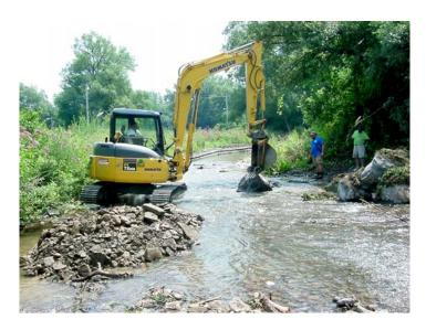
Using large rocks, a grade control structure is created, to prevent stream down cutting.
