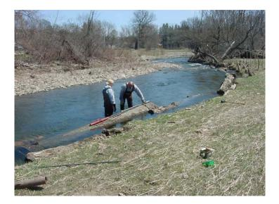
Anchoring revetments with duckbill anchors.
