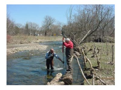
Driving duckbill anchors into streambed.
