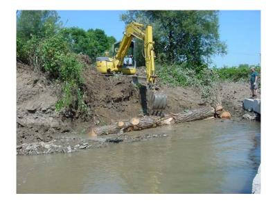
The excavator lowers the large tree trunks, which are then secured with cable to another log buried in the streambank.
