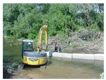
Concrete barriers are placed in the channel to divert the flow into the preexisting overflow channel during construction.
