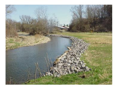
Stone placement complete to protect revetments.
