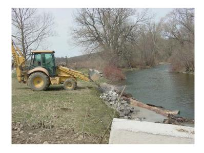
Installing stone behind revetments.
