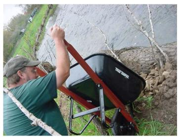
Placing rock behind revetments.
