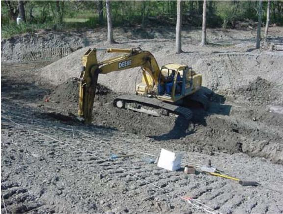
Trenches were dug at the base of the slope to install key logs into the bed of the stream.
