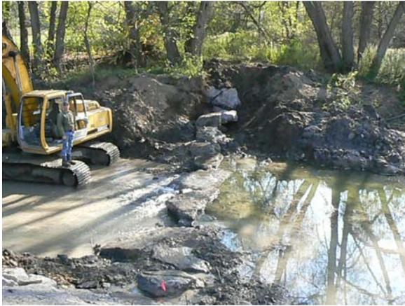
**Starting rock gradecontrol at end of slope rock and keyed into bank on east side of stream**
