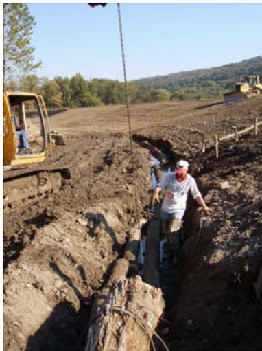
The excavator pulled and set the anchor in the stream to hold the key log down
