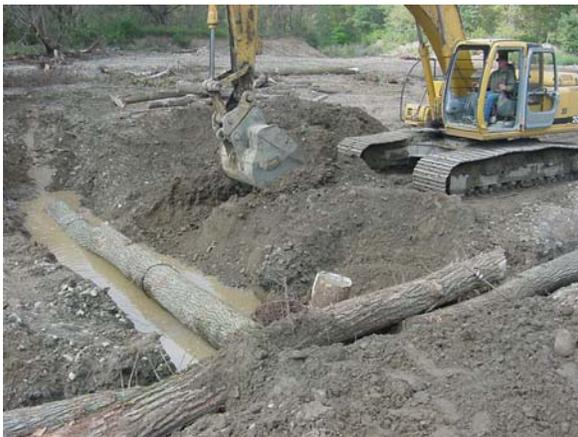
**Stumps were placed of the downstream side to further anchor the log and have sprouts come from the stumps**
