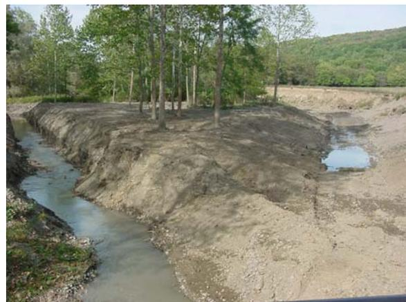
**Water diverted from work area so construction of revetments and grade controls can begin.**
