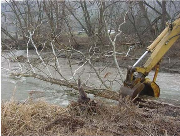
**Moving tree out of stream and using it for temporary bank stabilization above the bridge**
