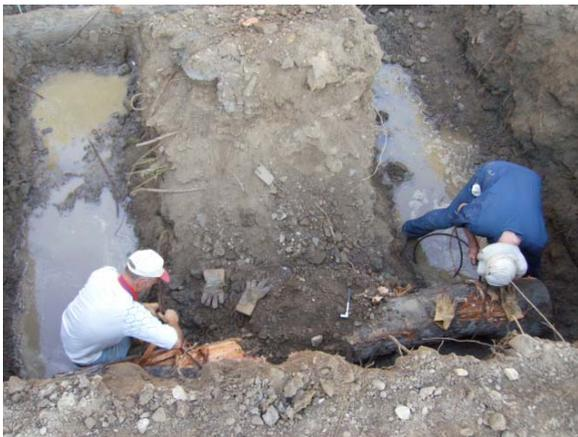
Cables were attached to the logs and later attached to the revetments to hold them in place
