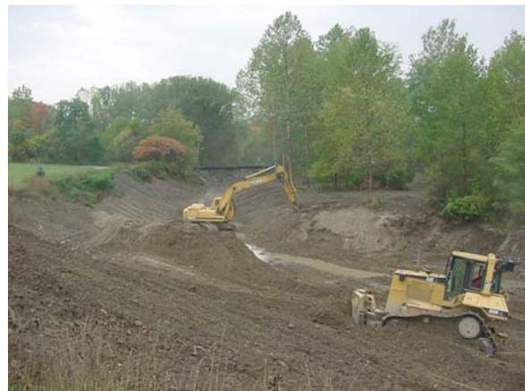
**It took the contractor one week to install diversion and grade the eroded bank for the revetments with so much material to move**
