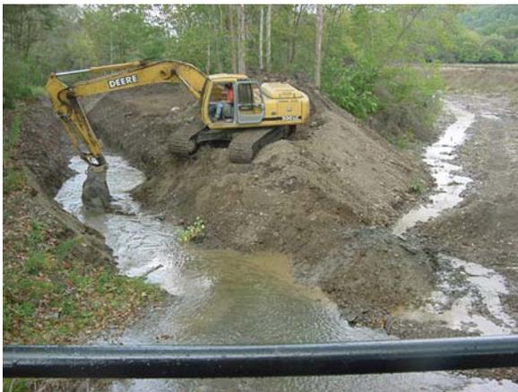
**Moving stream flow to new diversion channel**
