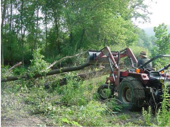
**Landowner helps SWCD staff dragging logs and poles to be used with log revetments**
