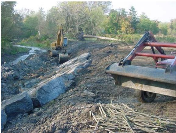
**Placing slope rock and placing planting between rock as required by permit**
