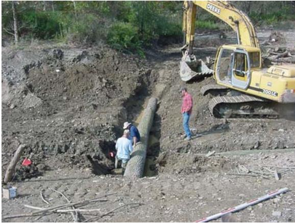
**A large log was used as a grade control at the midpoint in the log revetments**
