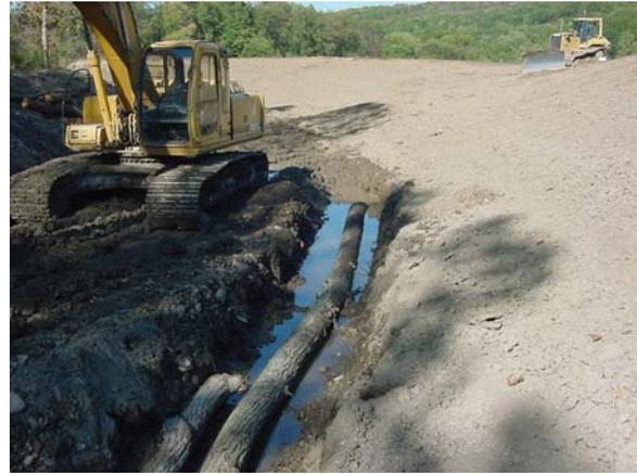
Key logs were placed in trenches and then logs were placed and cabled to the top of them
