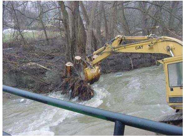
**Using stump to key in rock to protect bridge**
