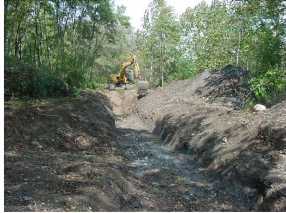
**Digging new diversion channel to divert water during project and to be used as an overflow channel after completion**
