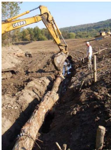
Logs were placed on top of key logs and cabled to the key log
