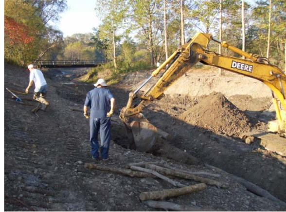
Logs were placed into the hole by the excavator
