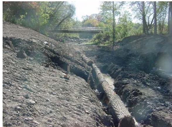
Logs after being placed together and logs were secured both with a duckbill anchor and a deadman in the bank
