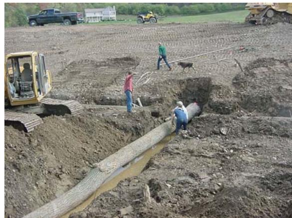
Then the cable of the duckbill anchor was cabled around the logs to hold them in place
