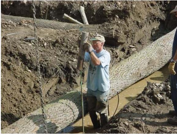
The duckbill anchor was driven into the streambed
