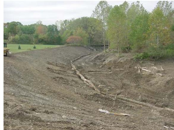
**View of revetments anchored in place ready for rock to protect from scour**
