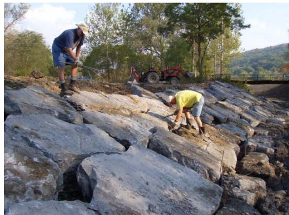
**Placing plantings on completed slope rock**
