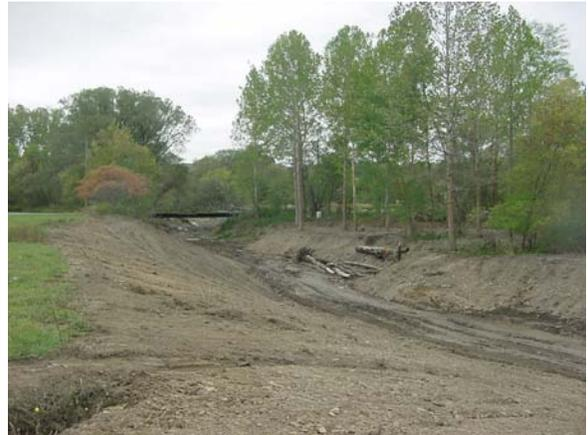
**Logs are placed near bank to be installed as revetments**
