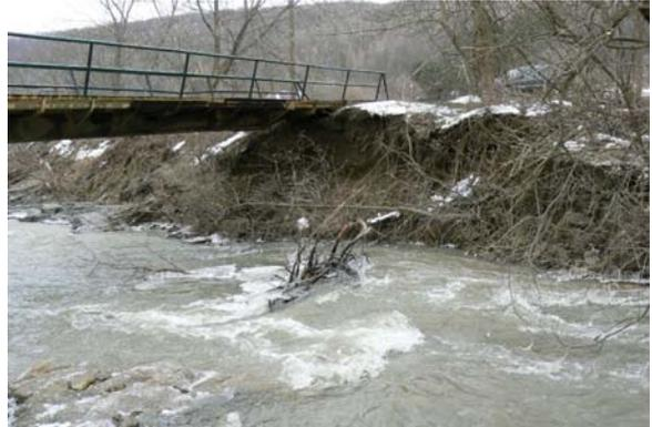
**Landowner bridge being under cut from resulting head cutting by stream due to blow out of lower meander**
