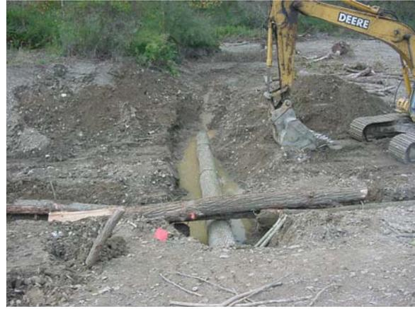
**The log was anchored in with the duck-bills and revetment logs were cabled on top to hold it in place**
