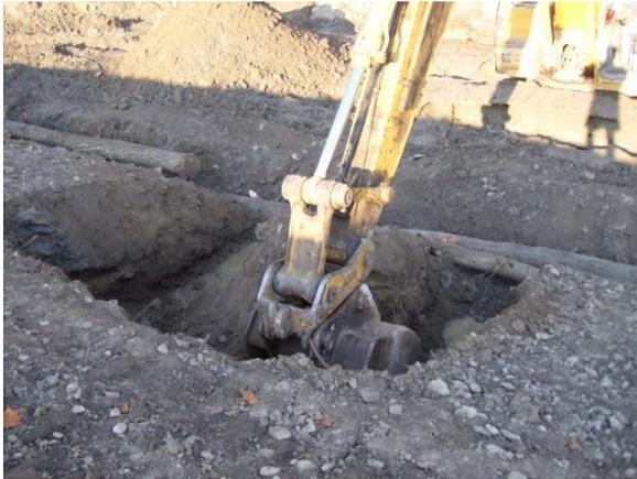
Holes were dug into the bank to place deadmen logs to hold in revetments
