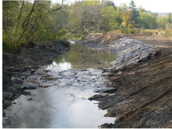
**Rock grade completed and end of slope rock**
