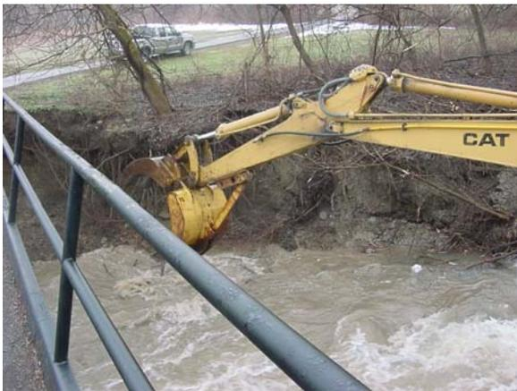
**Placing rock to save bridge in high water under emergency permit authorization**
