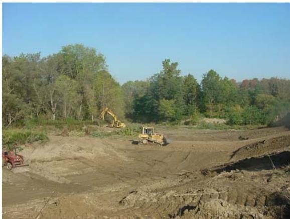
**Material was used from past runoff deposits to protect eroded bank now that the stream channel had been diverted**
