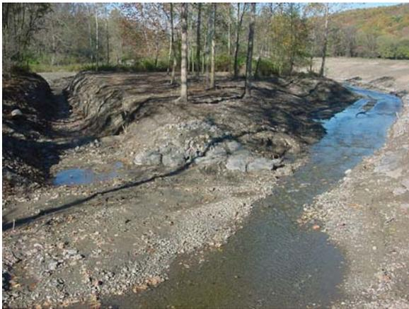
**Overflow diversion and new channel after complete**
