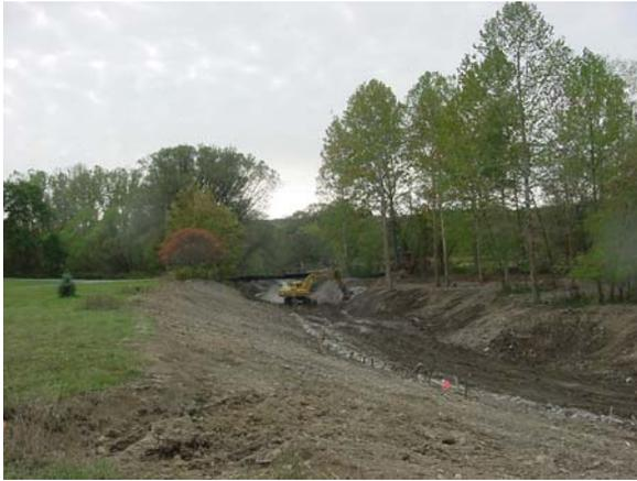
**Rock was placed by excavator and hand behind revetments to protect newly graded slope**
