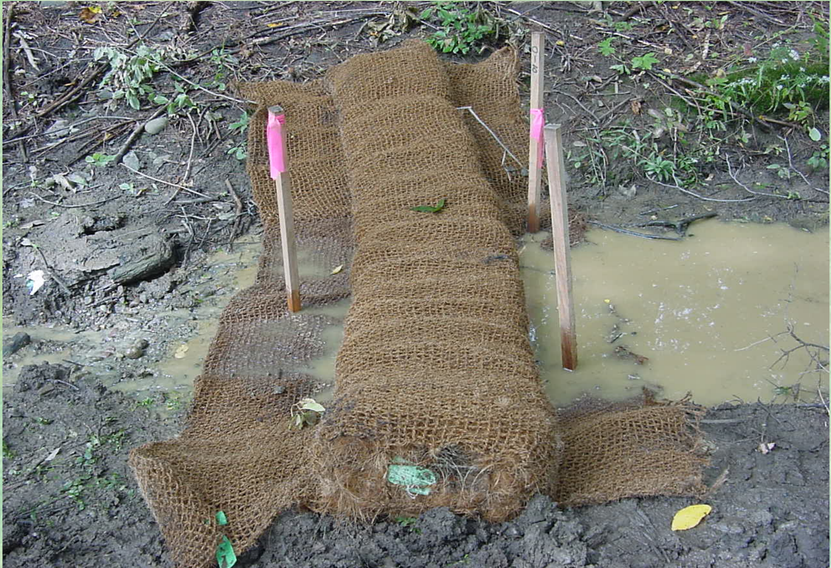
Coconut Fiber Coir Logs Installed as Permanent Check Dams
