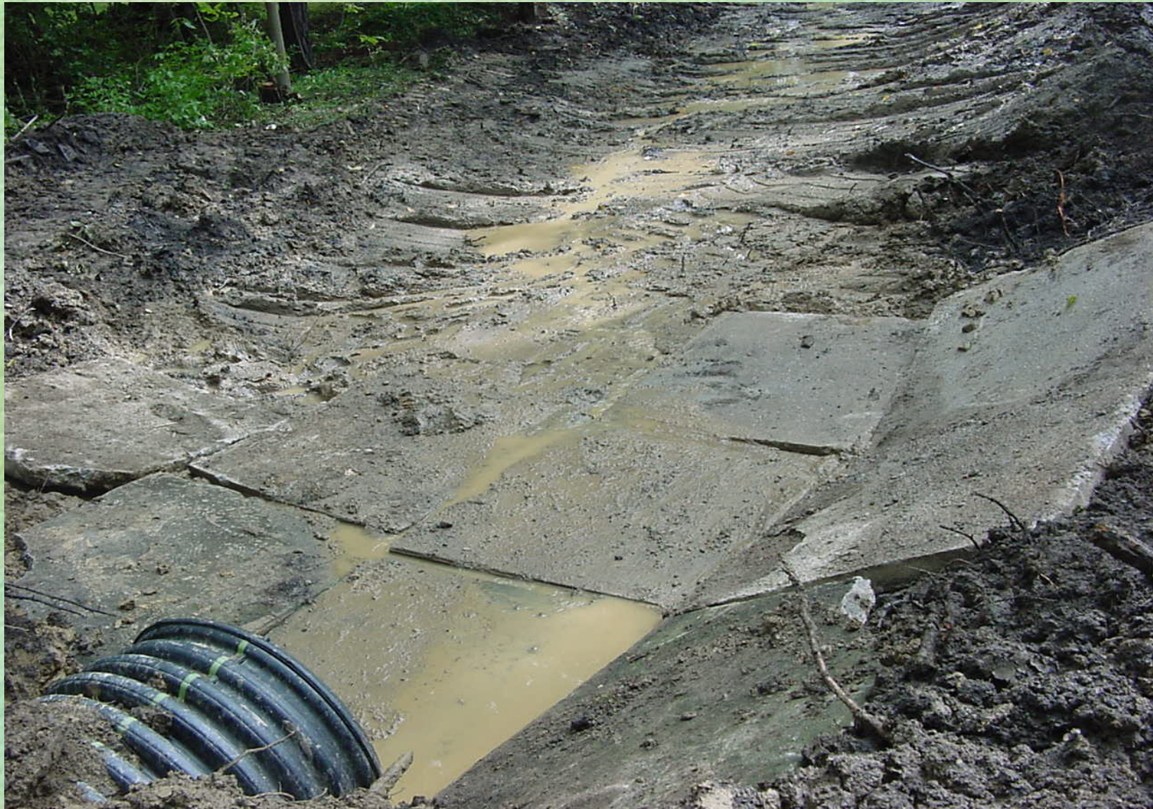
New 30'' plastic culvert pipe with outlet protection.
