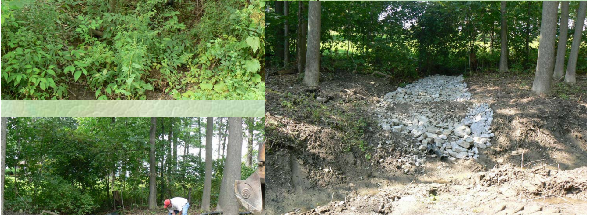
Repaired with Geotextile Fabric and Gabion Rock.
