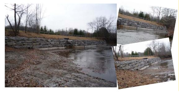
**Top Left** - Streambank stabilization to remediate an exposed water line in the Town of Attica, NY.
