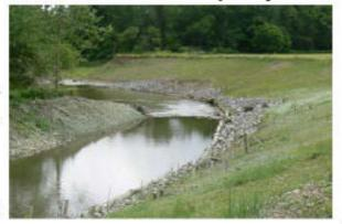
2 rock vane deflectors were installed. Trout Unlimited contributed to the project by planting trees for erosion control. The total cost of this project was \$68, 594.15.
