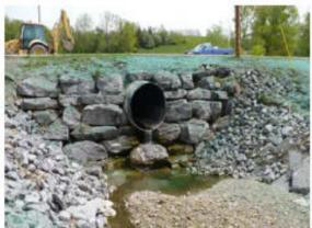
The project included the construction of a stacked rock wall and rock plunge pool, 2 rock cross vanes, and 50ft of riprap bank protection. Erosion
