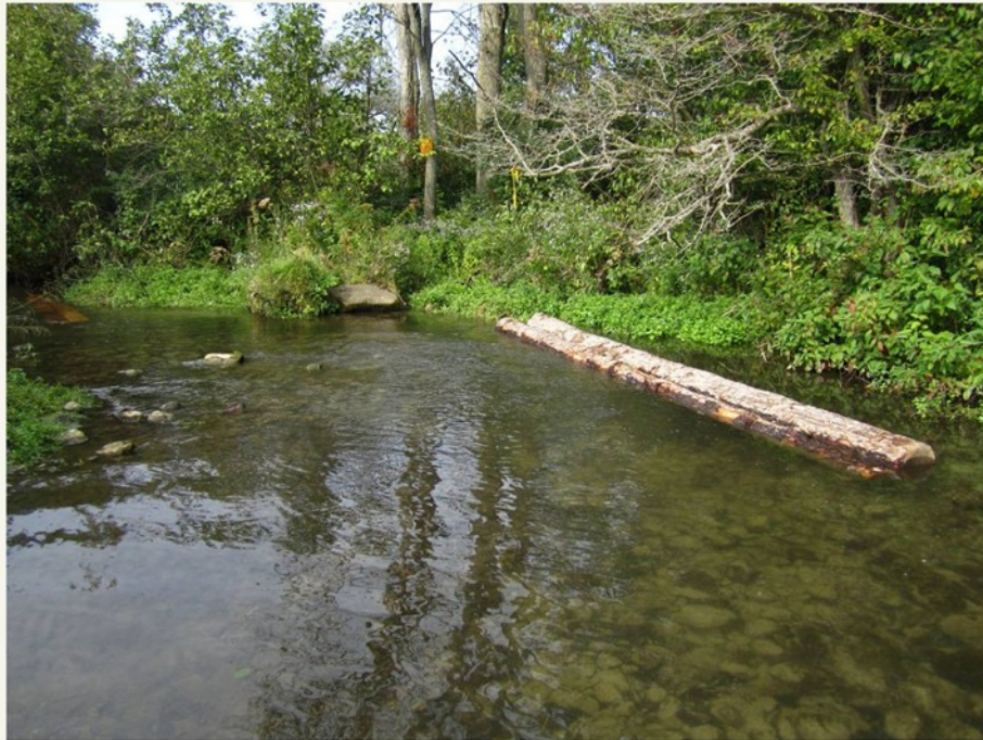
Figure 18. Cover logs installed on N. Branch.
