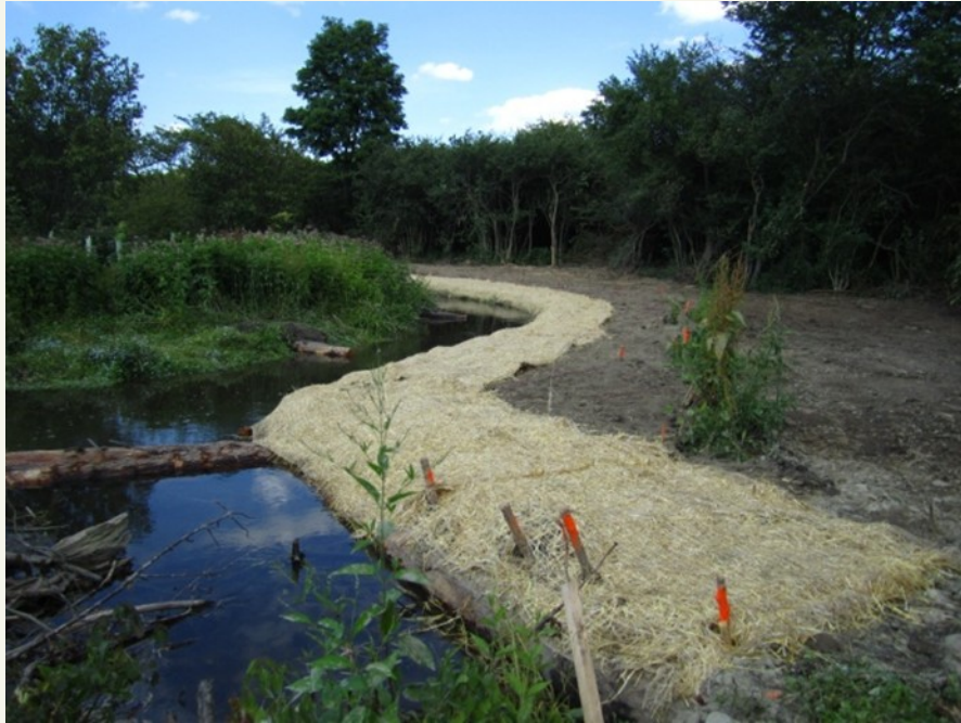
Figure 12. Erosion control blanket installed on LUNKERS.
