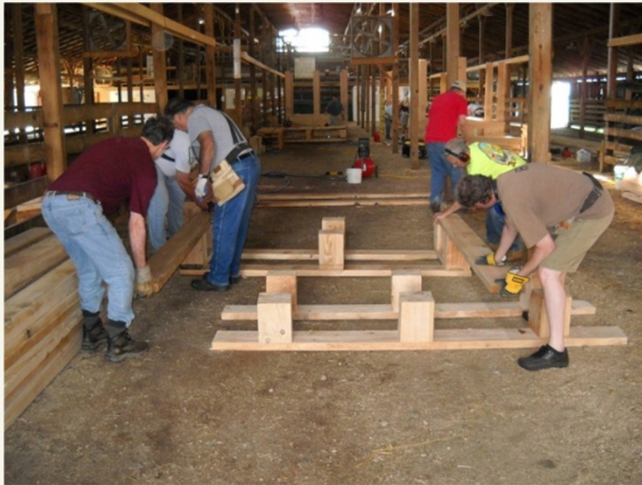
Figure 6. LUNKER construction at Wyoming County Fairgrounds by WNYTU volunteers.
