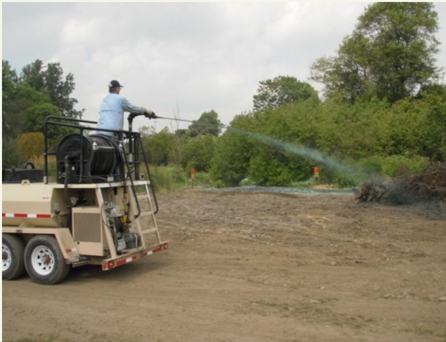
Figure 13. Wyoming Co. Highway Dept. hydroseeding and mulching.
