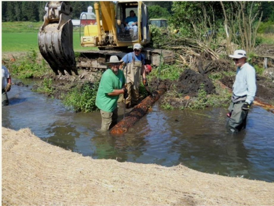
Figure 11. Installing a point bar log.
