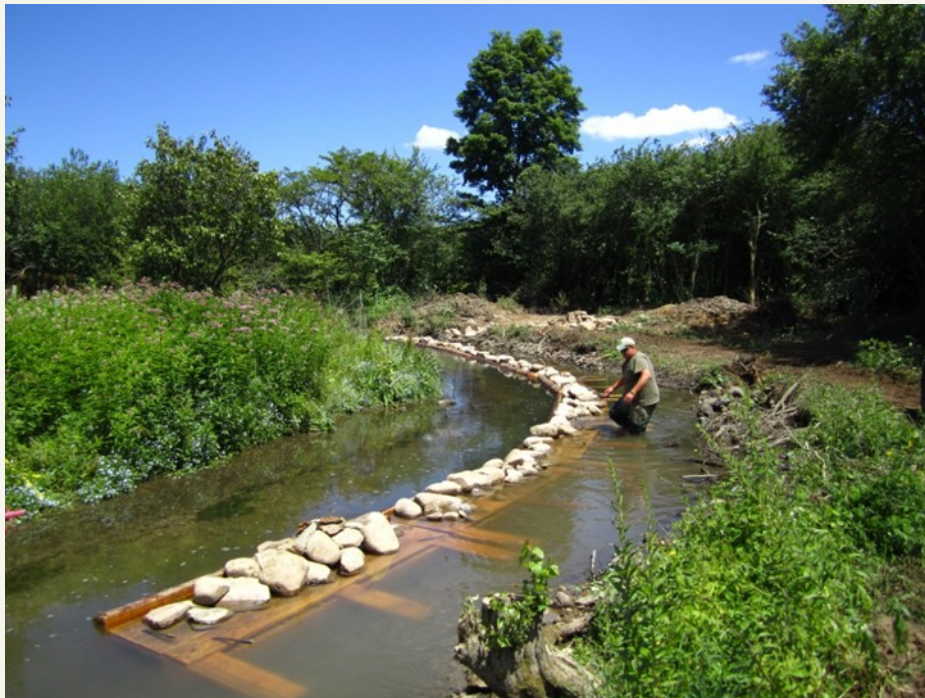
Figure 9. Hand placing heavy stone on LUNKERS.
