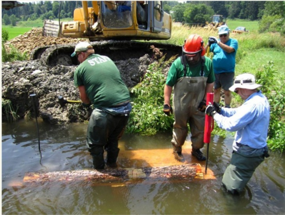
Figure 8. Hand driving rebar through a LUNKER.
