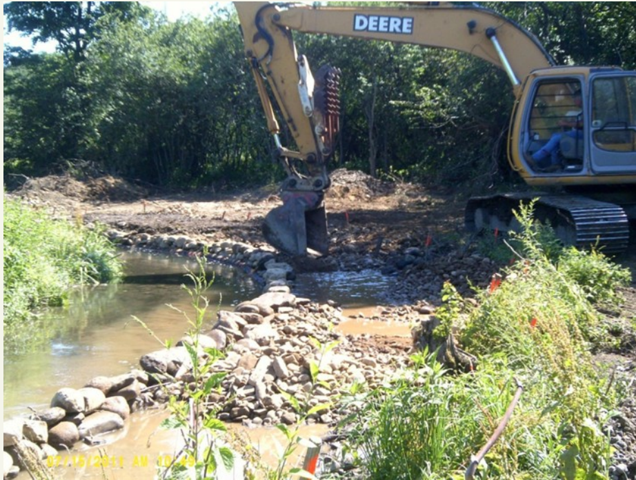
Figure 10. Back filling the LUNKERS.
