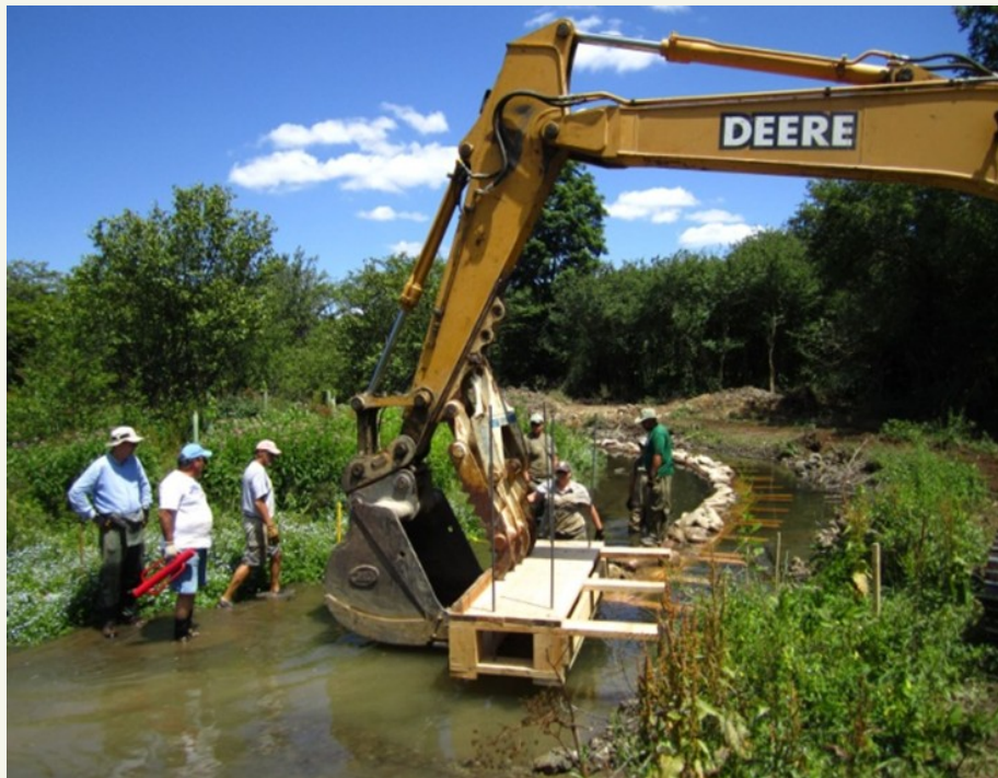
Figure 7. Excavator and volunteers placing LUNKERS at Site #6.
