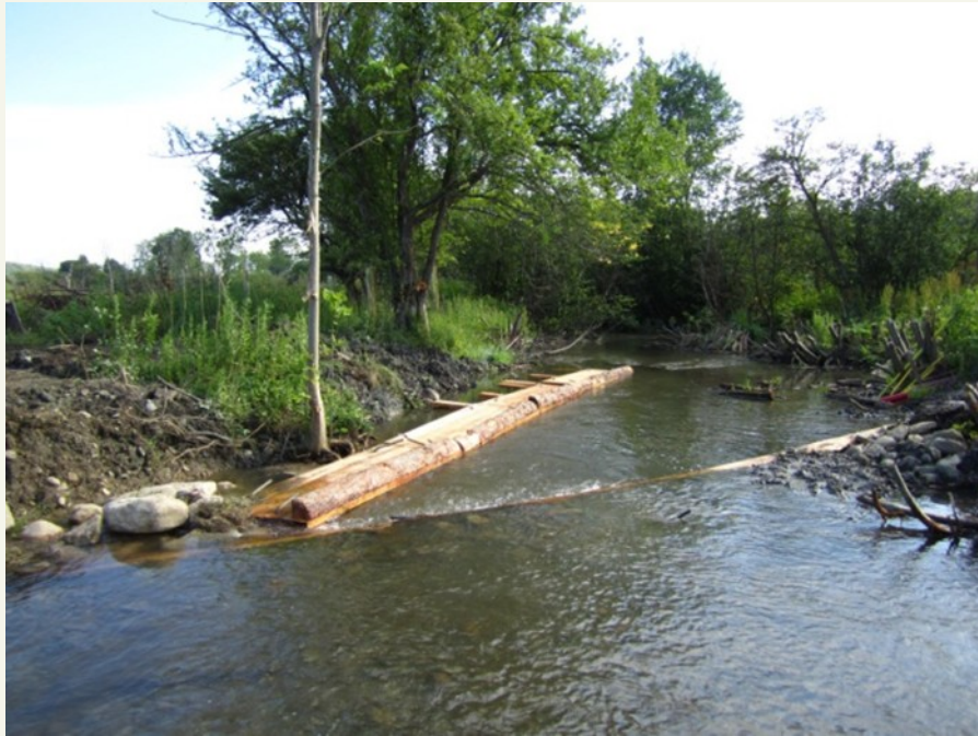
Figure 16. Partially constructed cross log with LUNKERS at Site #4.
