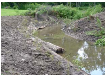
Log revetment at Mark McGrath Streambank
