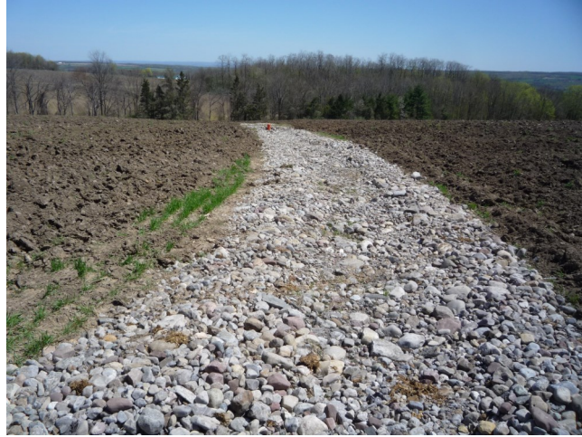
Completed rock-lined waterway at Harkins Dairy Farm.
