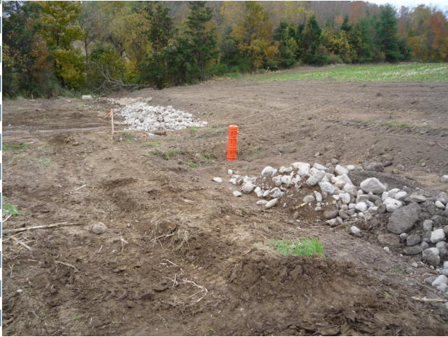
Water and sediment control basin with surface inlet at Harkins Dairy Farm.
