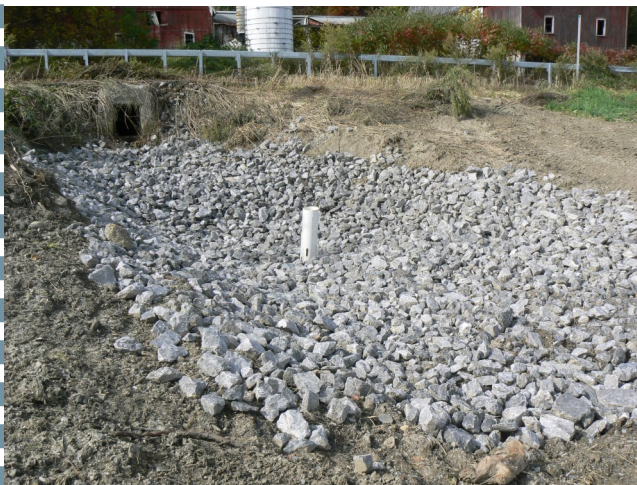
Rock-lined water and sediment control basin with surface inlet at the Jeffres Farm.
