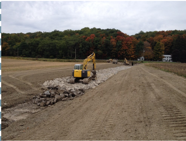
Rock-lined waterway under construction at R. L. Jeffres & Sons Farm.
