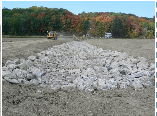
Completed rock-lined waterway at the Jeffres Farm.
