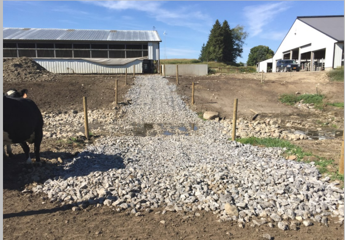
Stoney Creek Farm, LLC Cattle Crossings/Livestock Exclusion Fencing
