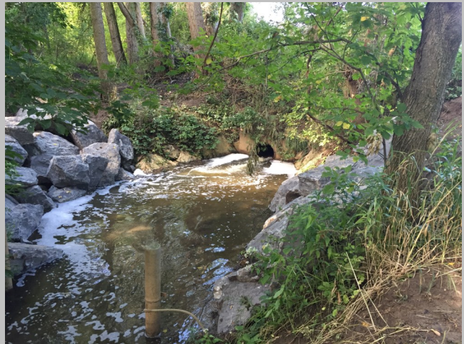
Attica WWTP Stream Stabilization - After
