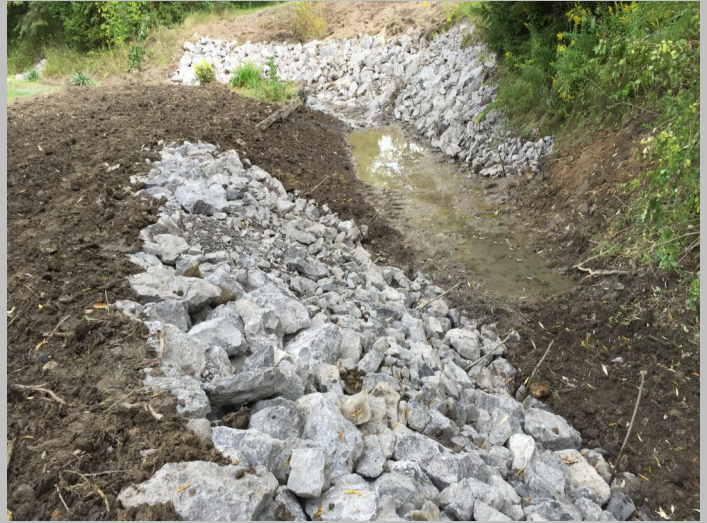
Tributary of Tonawanda Creek Streambank Stabilization in the Town of Sheldon - FEMA Project
