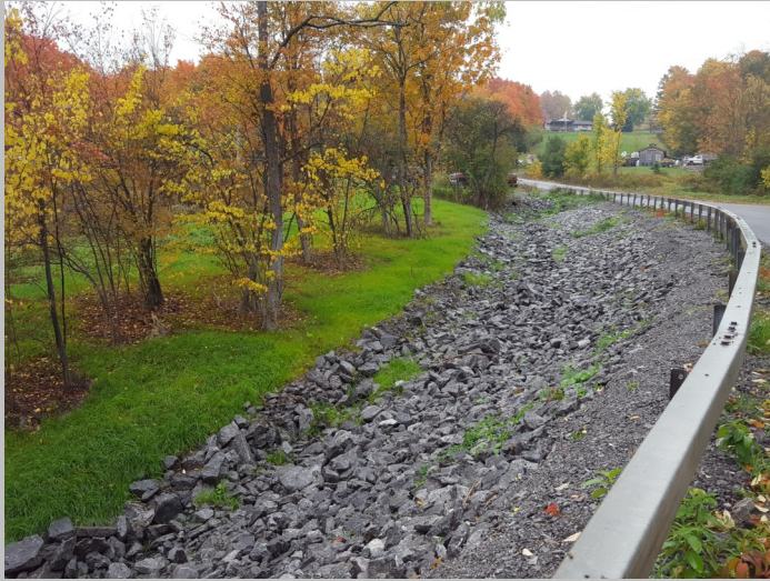
Merkle Road Streambank Stabilization in the Town of Attica - FEMA Project
