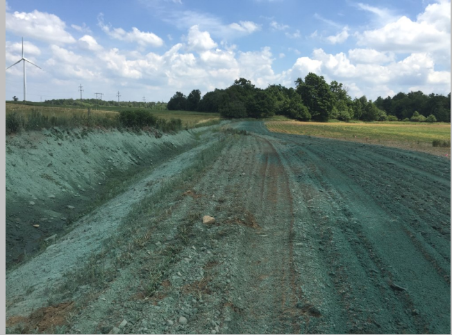
Hydroseeding at Fugle Dairy Farm
