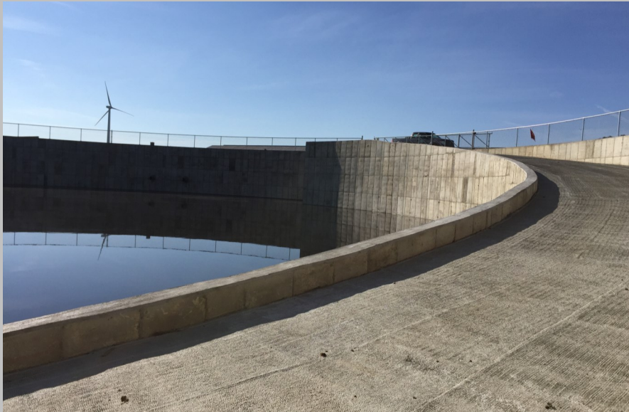
Construction of Waste Storage at Davis Valley Farm, LLC
