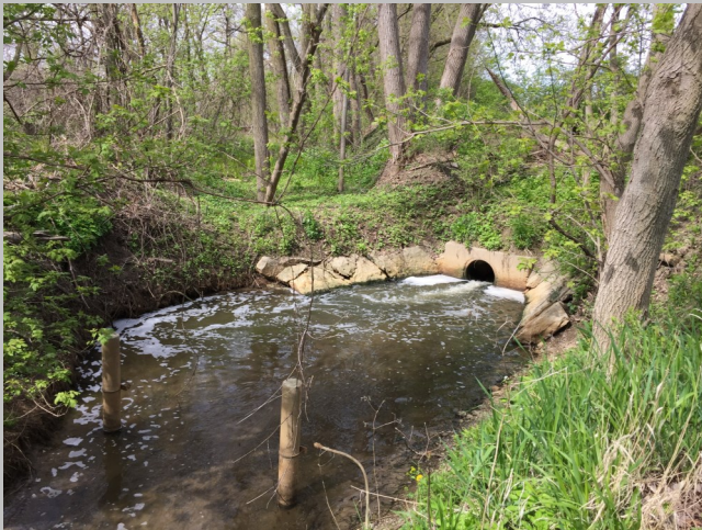
Attica WWTP Stream Stabilization - Before
