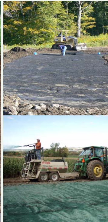
Lining waterway with geotextile fabric and hydroseeding
