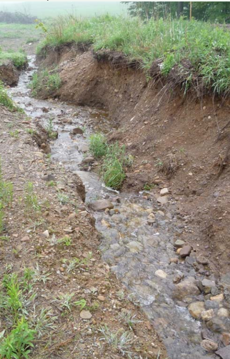
Erosion problems before
