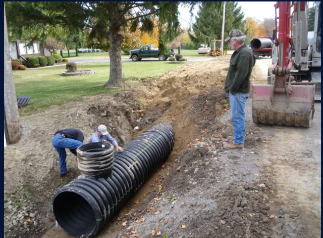
Town of Castile, Club Road Stabilization Project
