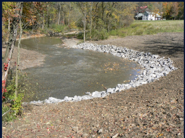
Wyoming/Erie County Joint Board Buffalo Creek, Streambank Stabilization
