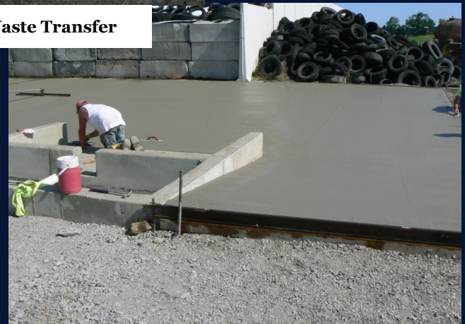
Fontaine Farms, Silage Leachate Management System
