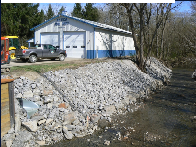
Village of Attica, Streambank Stabilization
