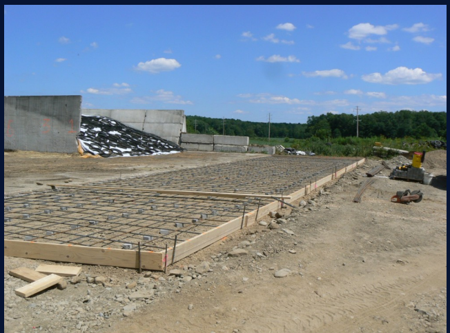
Zielenieski Farms, Silage Leachate Management System
