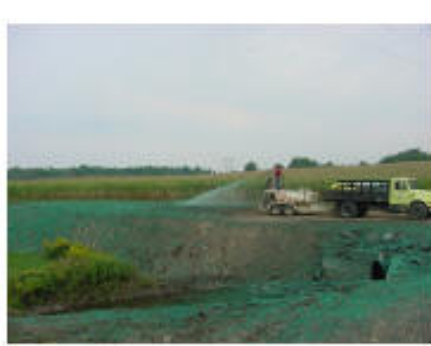
Hydroseeding at Bacon Rd.
