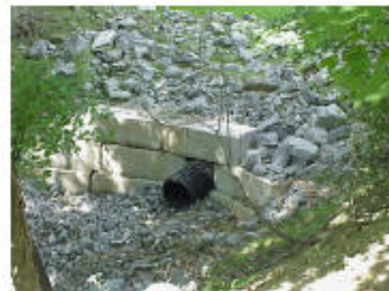
New Culvert on Cornwell Rd.
