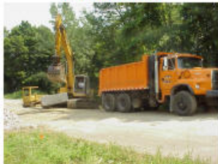
Construction at Cornwell Rd.
